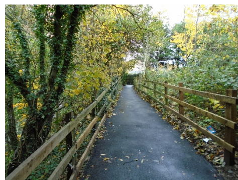
New footpath surface near Lanelay Park
